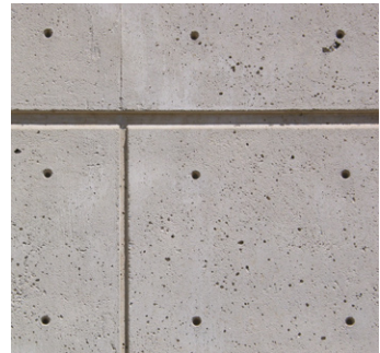
POURED-IN-PLACE CONCRETE POULTRY SCIENCE
