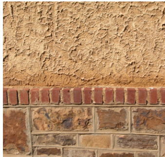
STUCCO OLD WOMEN'S GYMNASIUM
