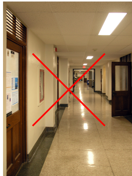
fluorescent lights, drop-in ceiling, etc. circa 1990
