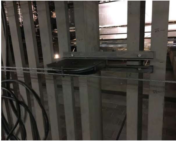
The images above show cables rubbing on loft blocks.
