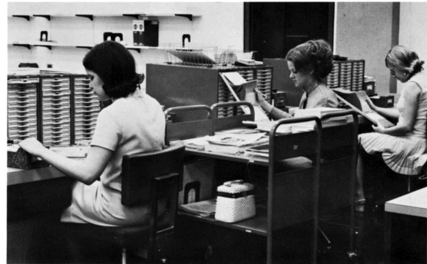
Serials receiving section where magazines are received, recorded and distributed to various areas in the Library.
