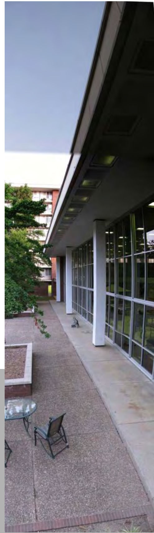
East Façade – A Wing
