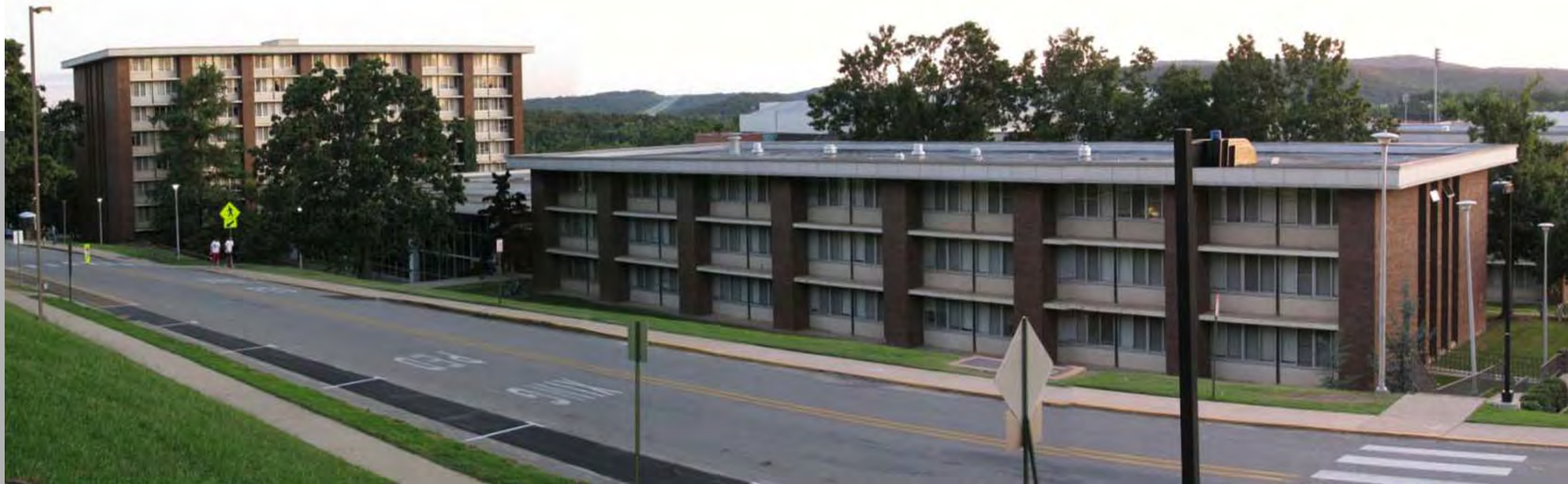
East Façade of Building
