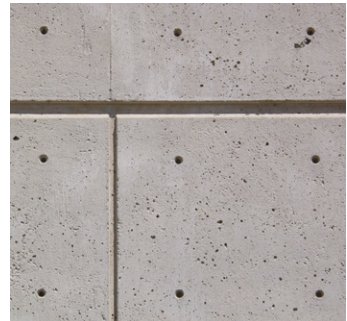
POURED-IN-PLACE CONCRETE POULTRY SCIENCE
