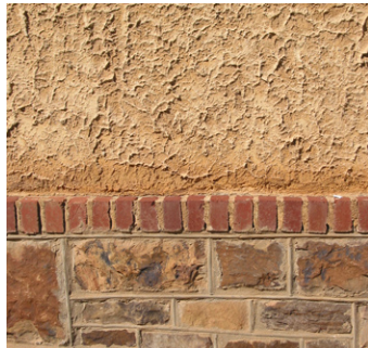
STUCCO OLD WOMEN'S GYMNASIUM
