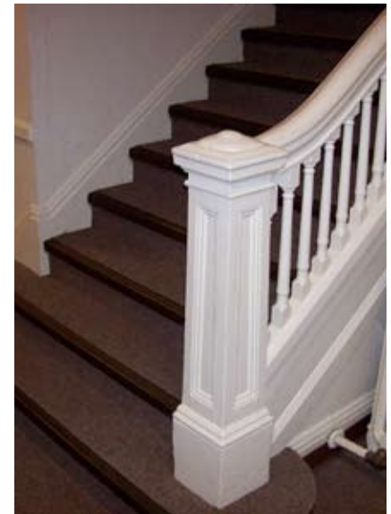
Figure 105. Interior features such as historic stairs, baseboards, doors, ceiling and floor finishes can be preserved as part of reuse strategies. This image shows a historic stair newel post in the Academic Support Building. Concealing historic features by installing drop ceilings or other means should be avoided.
