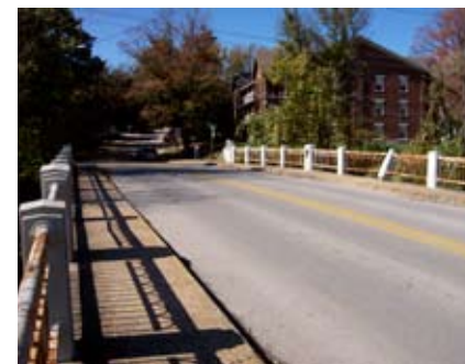
Figure 56. View of West Lafayette Street overpass.
