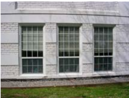
Figure 89. The replacement window units installed at Peabody Hall are comprised of single panes of glass with applied muntins. This approach does not capture the subtle characteristics of the original windows.
