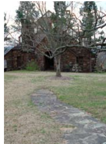
Figure 83. Restoration of the McLroy House landscape should be given consideration.
