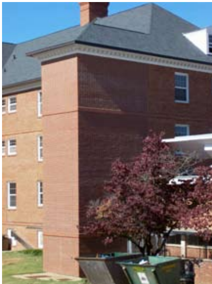
Figure 100. In some cases it is necessary to modify the building exterior to incorporate means of access as seen here at Holcombe Hall. Where this is necessary, the guidelines for adding to historic structures should be followed.
