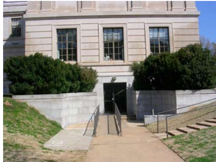
Figure 101. Accessibility to Vol Walker Hall is addressed in a number of ways. In this case access to the basement level is achieved by modifying the grade in this area of the building.
