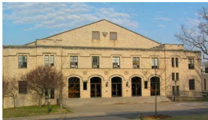
Figure 92. The installation of bronze-colored aluminum fully-glazed doors has altered the historic character of the former Men's Gymnasium.
