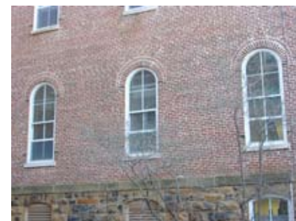
Figure 91. Storm windows have been installed on Old Main, increasing the building's energy efficiency and protecting the historic wood windows.
