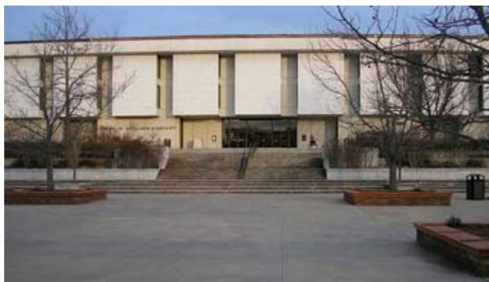
Figure 44. Current view of Mullins Library
