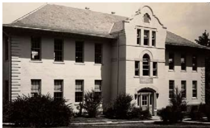
Figure 58. Historic view of Chemistry Building with its original Spanish Revival Style gable parapet over front entry bay.
