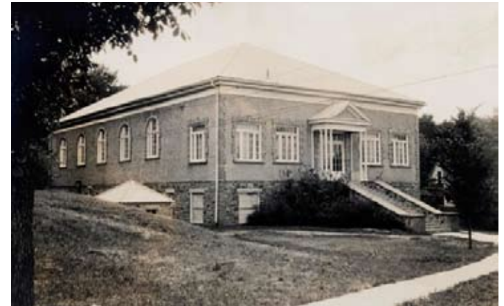
Figure 16. Women's Gymnasium/Army ROTC Building
