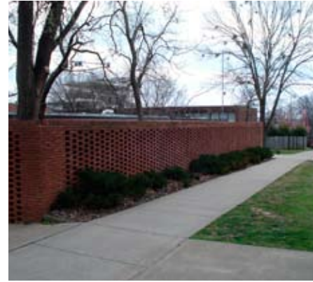
Pierced brick screen wall
