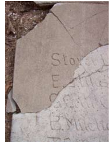
Figure 84. The oldest sections of the Senior Walk suffer from deterioration. View of concrete patch.
