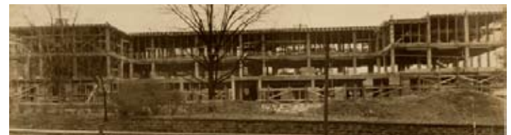
Figure 23. Photograph of Engineering Hall taken during construction.
