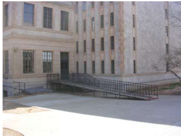
Figure 102. A less deliberate and more temporary approach to accessibility is taken at the rear entrance to Vol Walker Hall.
