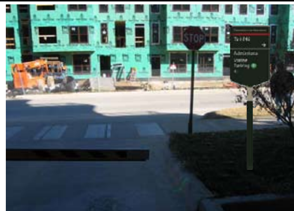
Sign illustrated in the photo does not contain actual message(s). See message schedule for actual sign content.
