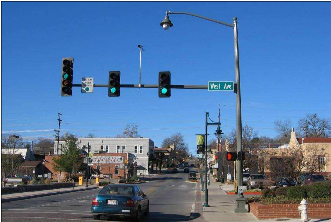
Photo 2: Dickson Street, looking west from West Avenue
