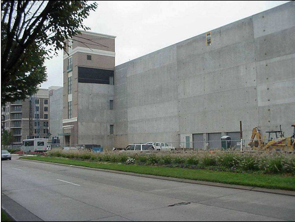
Photo 4: A deck with little architectural treatment, awaiting a wrap
