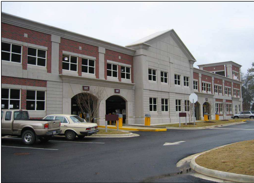
Photo 3: Example of a deck with extensive architectural treatment
