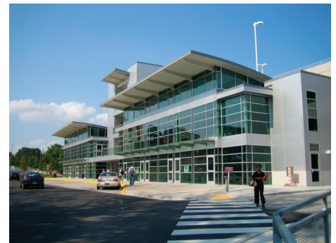
Recently completed Harmon Avenue Parking Facility
